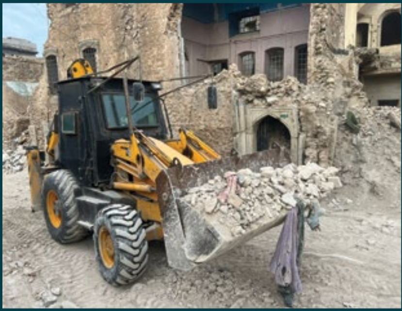
Tetra Tech clears rubble in Old Mosul, April 2023. Courtesy of Tetra Tech.
